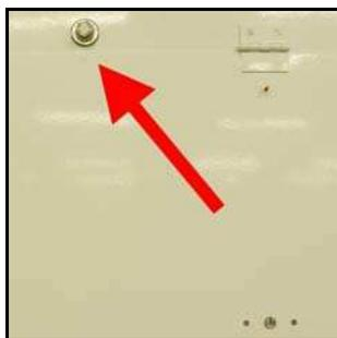
Figure 21 single measure point downstream exhaust HEPA filter
